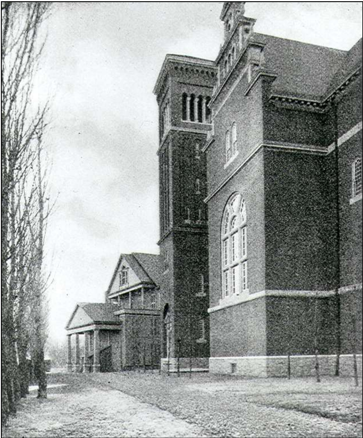
Serlo Organ Hall and the Methuen Organ Company factory building photographed looking southerly on Broadway around 1900.
